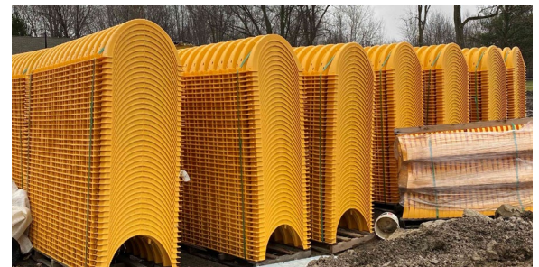
Future stormwater retention system
